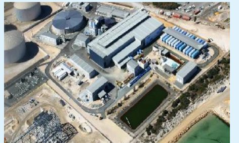
Perth Desalination Plant (Australia)
